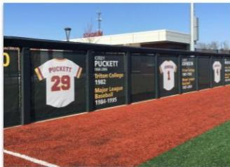
Custom padding panels are made of 3 inch thick polyurethane foam glued to a  $\frac{1}{4}$  inch treated plywood backer and covered with an 18 oz. vinyl covering, a coated UV polyester fabric.
