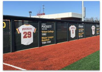
Custom padding panels are made of 3 inch thick polyurethane foam glued to a ¾ inch treated plywood backer and covered with an 18 oz. vinyl covering. Vinyl cover coated UV polyester fabric.
