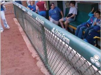
Panels shall consist of 3 inch thick polyurethane foam glued to a ¾ inch treated plywood backer and covered with an 18 oz. vinyl covering. Vinyl cover shall be coated UV polyester fabric.
